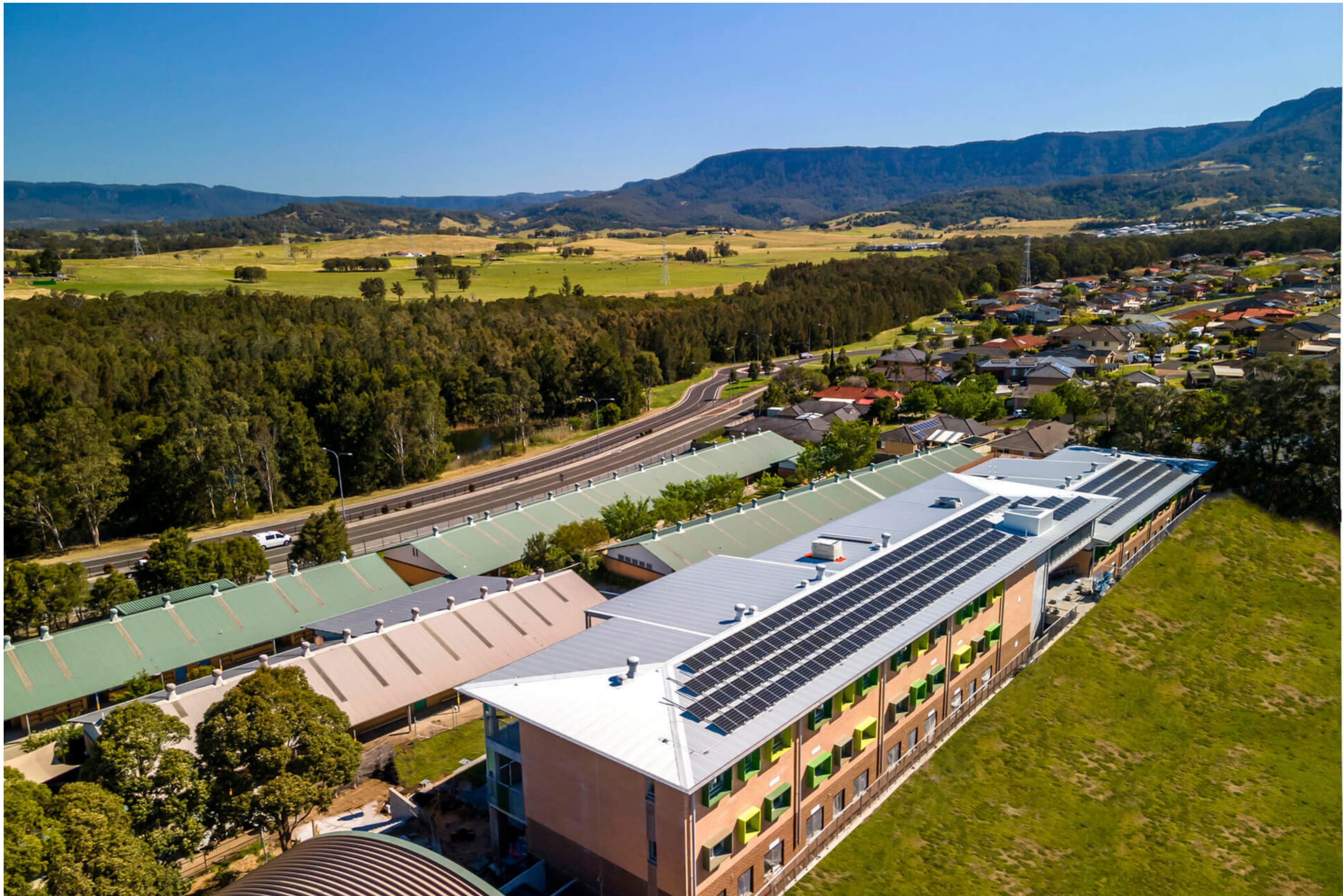
Source: Patterson Building Group
