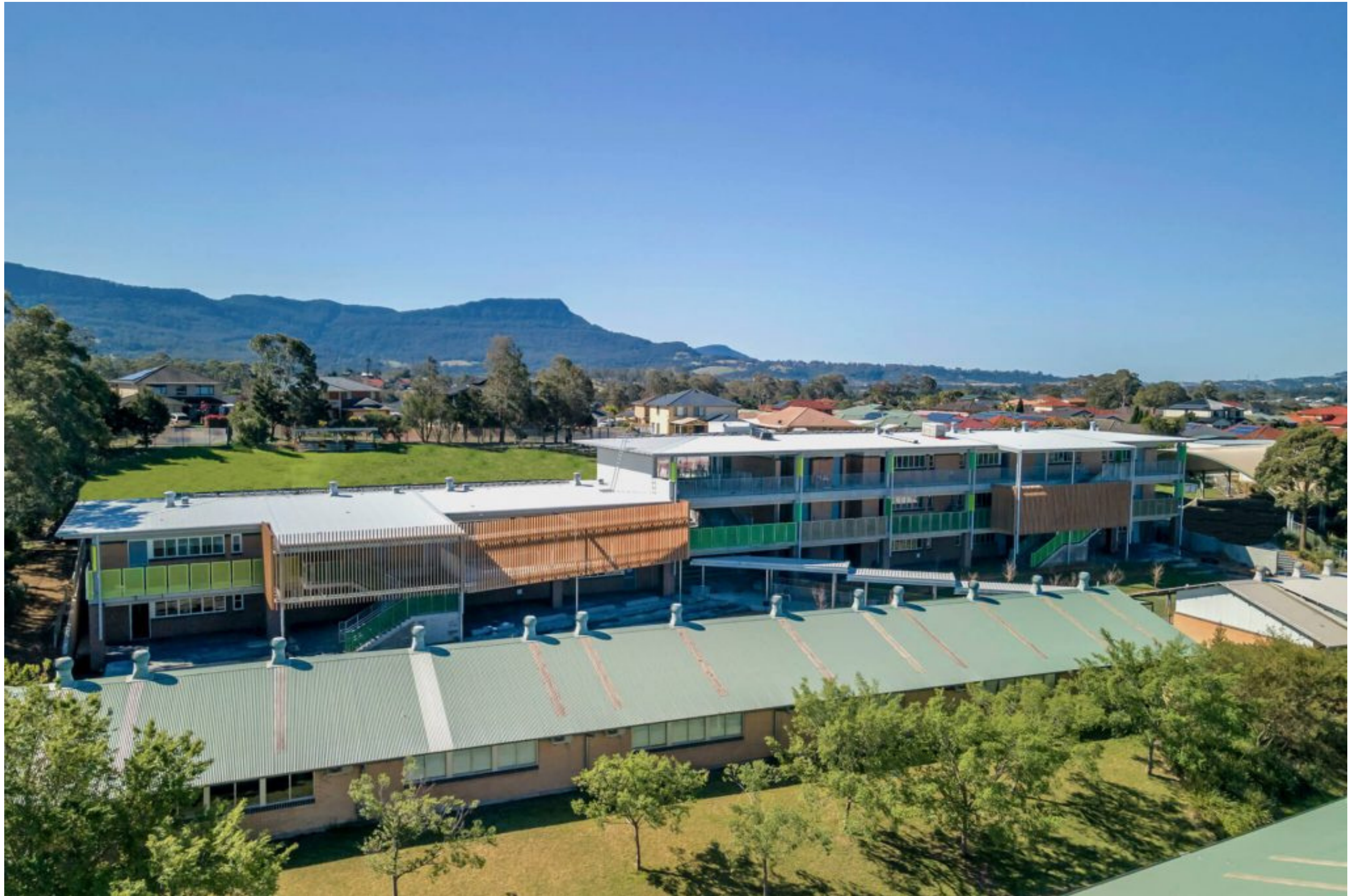
Source: Patterson Building Group
