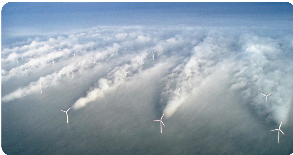
A light fog reveals the wake effect behind turbines at Vattenfall's Horns Rev wind farm off Denmark. Source: Recharge News
