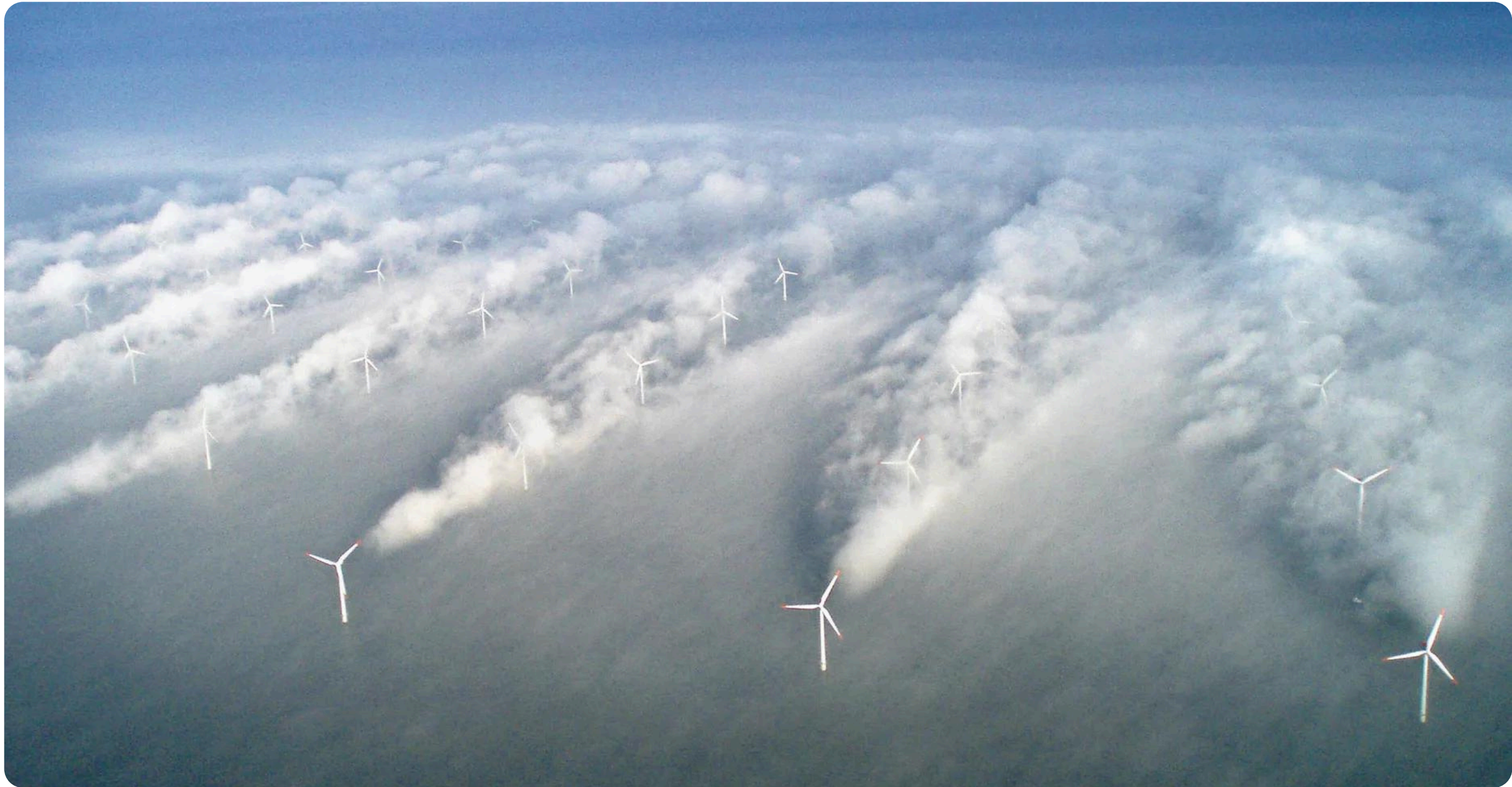
A light fog reveals the wake effect behind turbines at Vattenfall's Horns Rev Offshore wind farm off Denmark. Source: Recharge News
